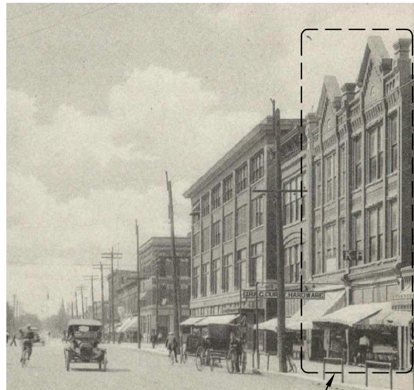
HISTORIC PHOTOGRAPH SHOWING ORNATE PARAPET, DOUBLE-HUNG WINDOWS, TRANSOMS ABOVE STOREFRONTS, AND AWNINGS
